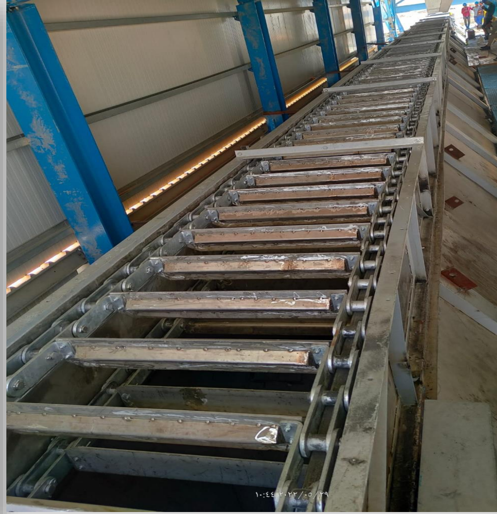
Final Sugar Drag station – W=1 m & L = 40 m
