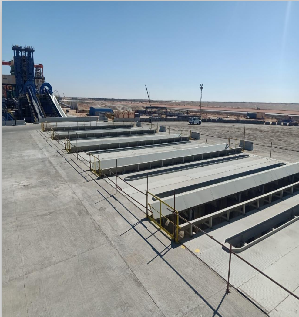
Tipping station “Biggest in the world” Consist of 10 fixed platforms / 6 movable platforms
