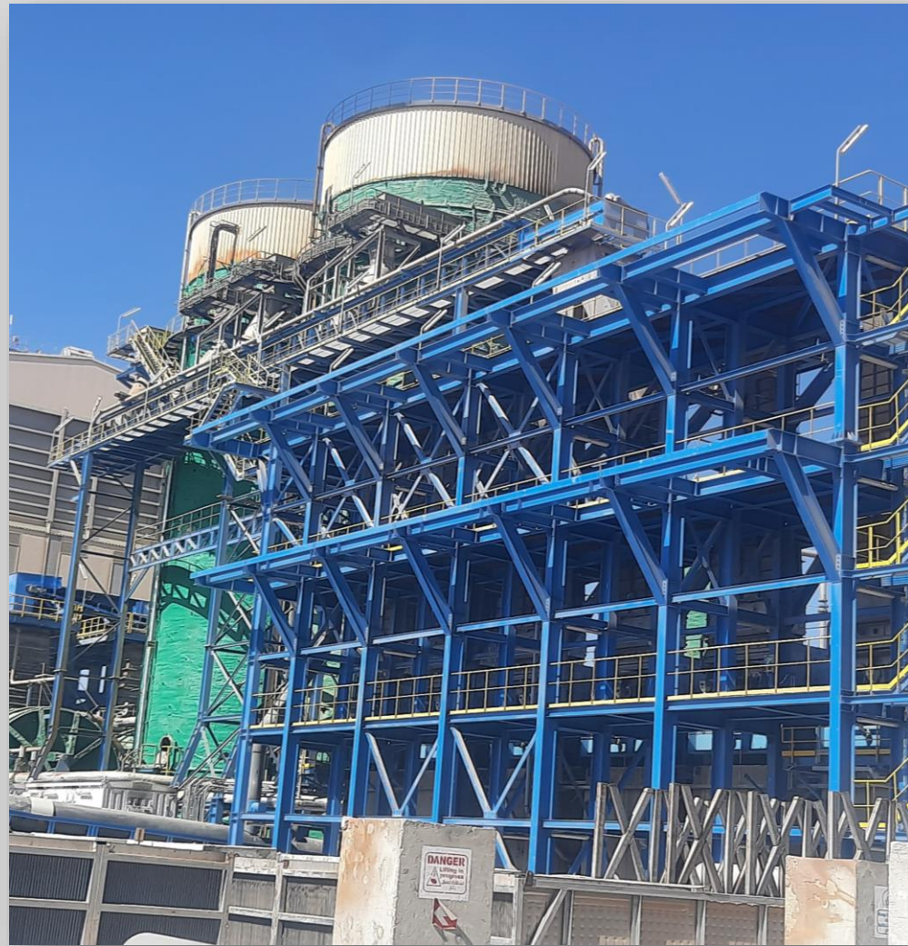
Pressed pulp station “Biggest in the world” Width 12m X Length 65m X Height 25m
