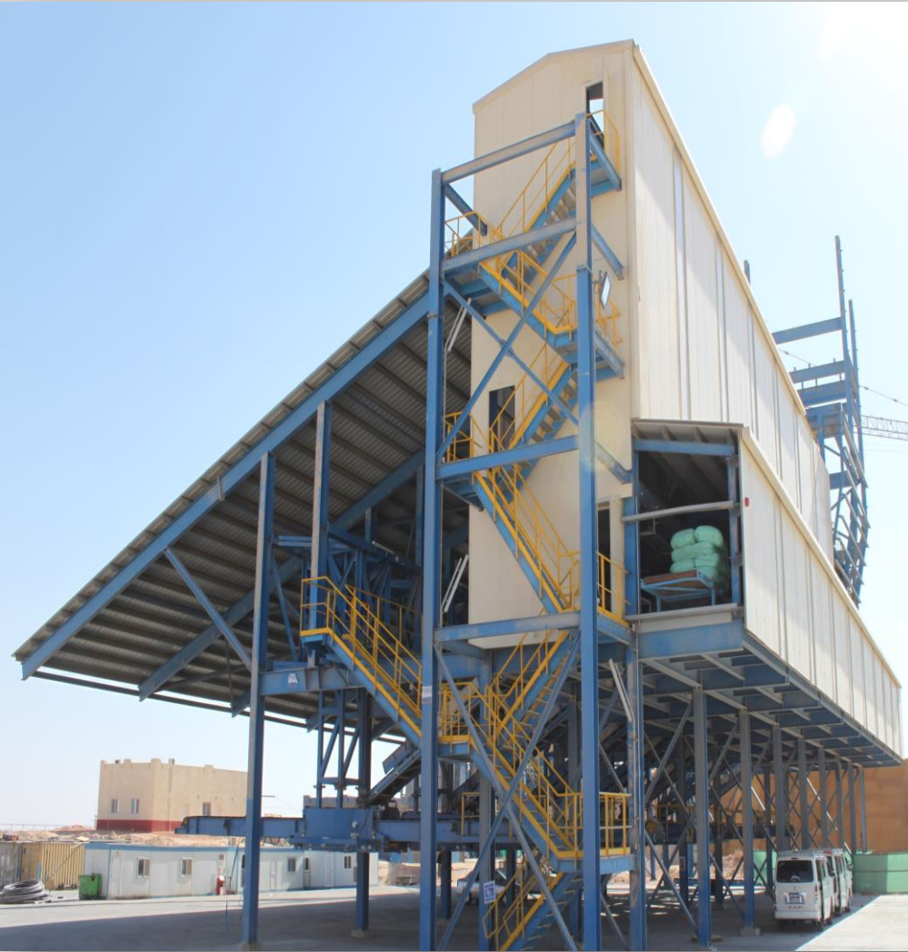
Bagging station “ Biggest in the world ” 8 bagging lines Width 30m X Length 75m X Height 40m
