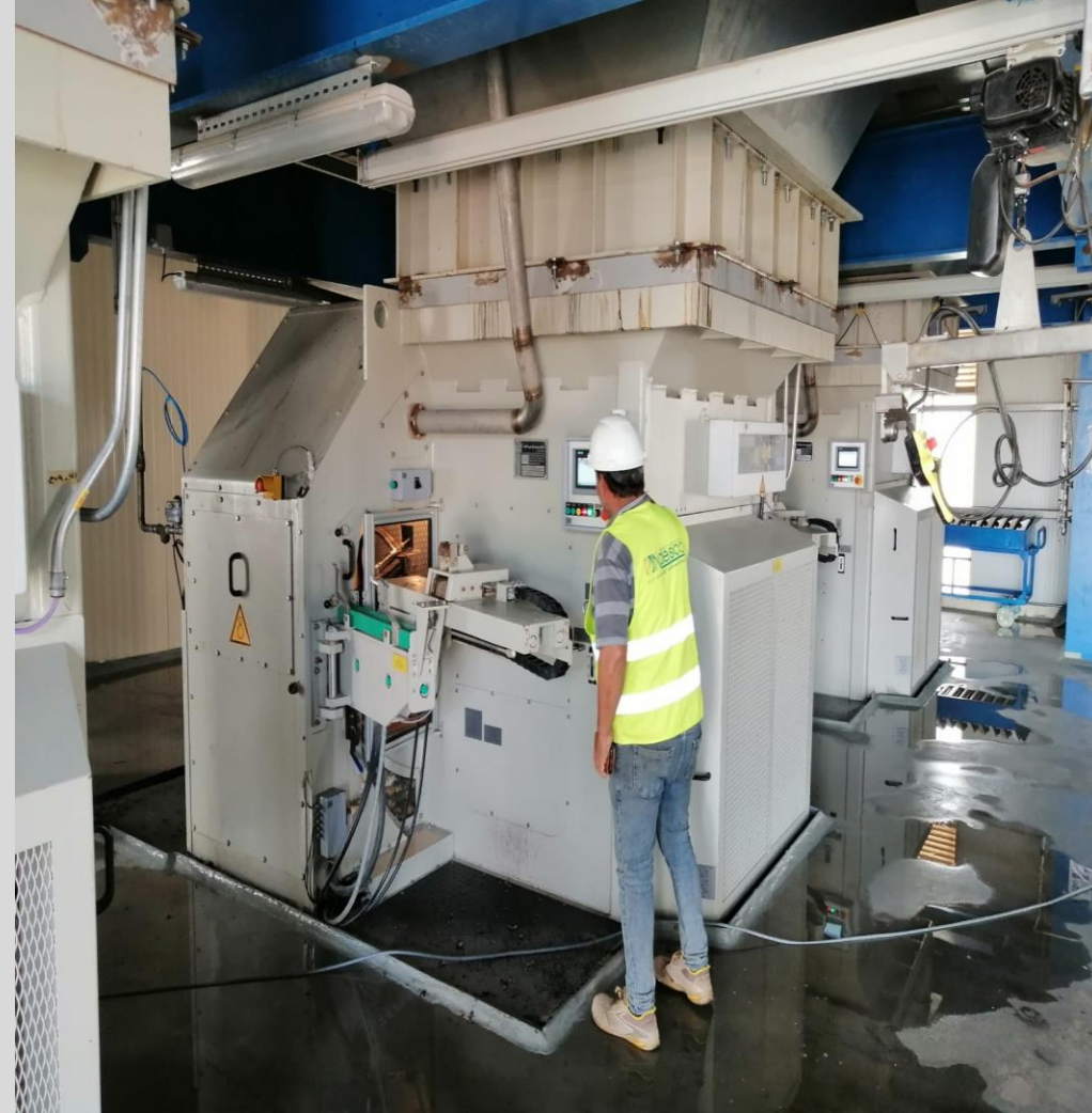
Clean beet bucket elevator “Biggest in the world” Capacity 1,500 Ton / Hr.
