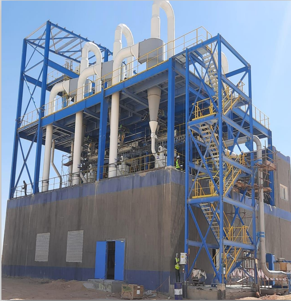
Pelletizing station (5 Pellet lines) Width 20m X Length 35m X Height 25m
