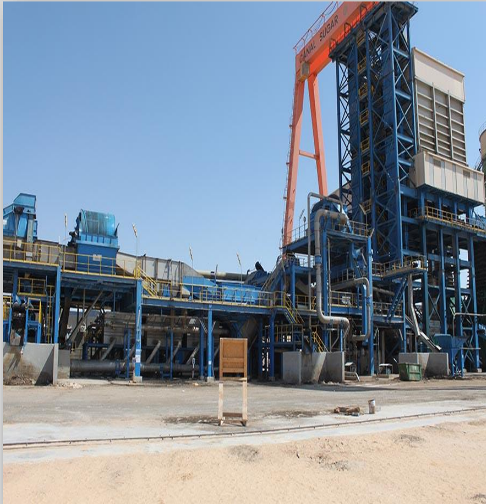
Slicing station “Biggest in the world” Width 25m X Length 40m X Height 40m
